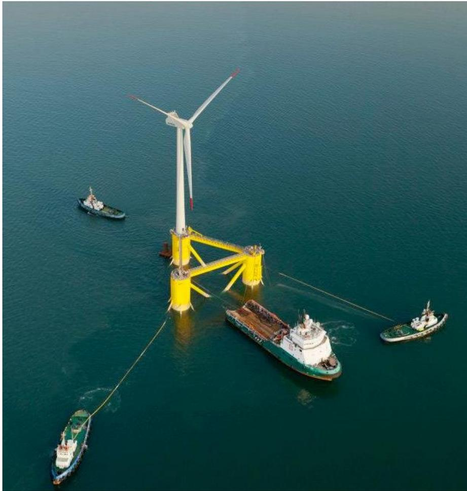
**Figure 6-5 Installation using towboat [WindFloat project]**
