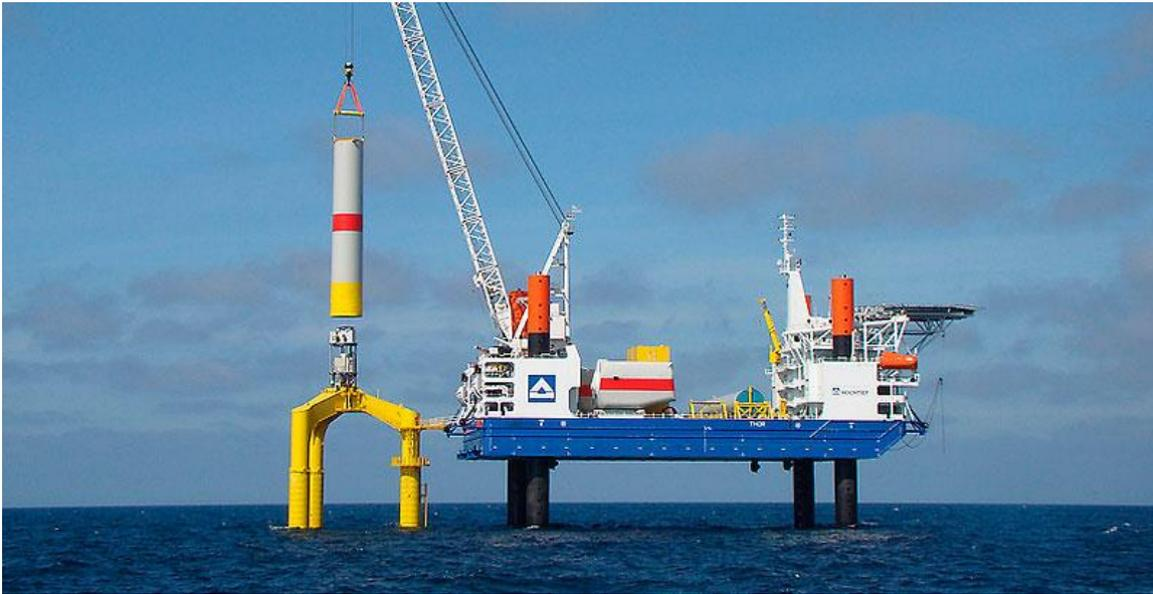
Figure 6-2 Installation on tri-pod type platform
