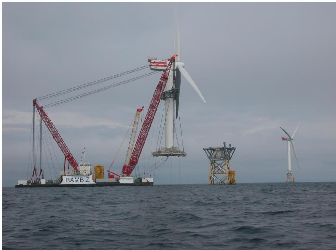
Figure 6-1 Installation on Jacket type platform
